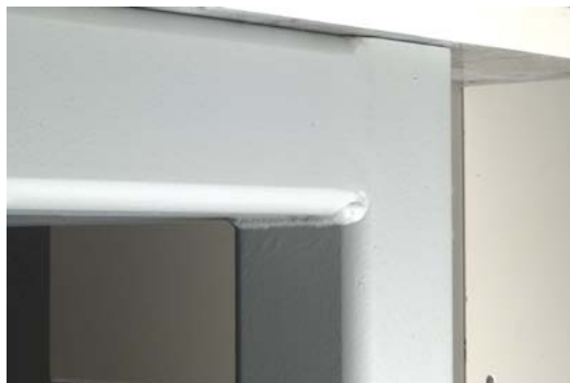
Welded Steel Frame Construction
